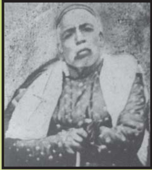
Late Padmadutt Balutiya Nainital
